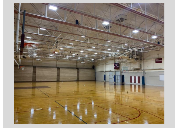
Chippewa Gymnasium LED Lighting
